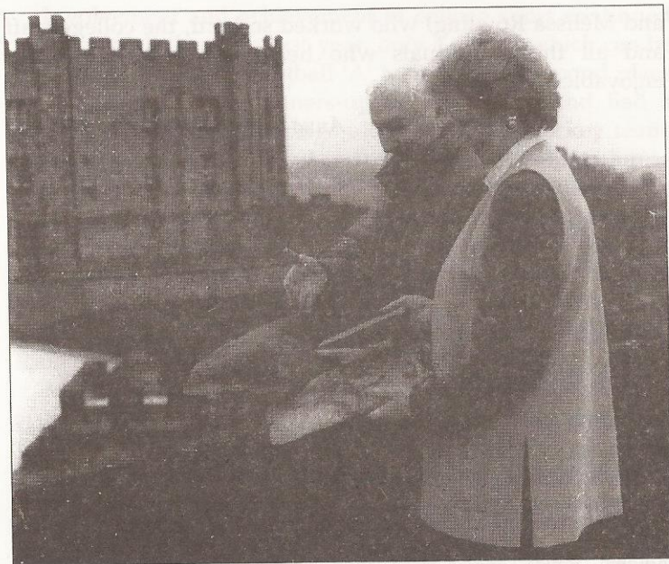
Our picture shows NAFAS Area Chairman, Mrs. Winn Alderslade, one of the organisers, looking at the structural problems the fund-raising has helped, upon the roof of the Castle with the Bursar, Wing Commander Albert Cartmell.
